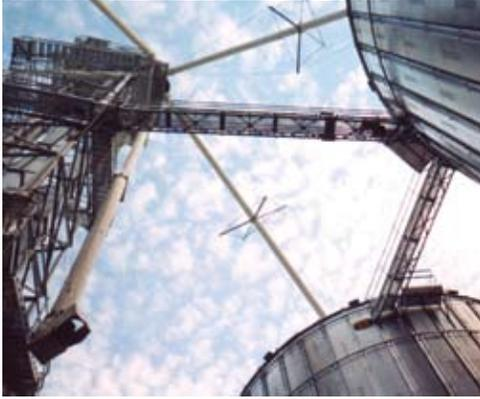
A pre-engineered galvanized modular conveyor support system with parallel walkway. Standard 20, 15, 10, and 5 foot sections afford fast and simple field erection with no on-site cutting or welding. Free spans to 100'.
